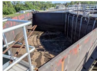
Figure 7: Plant 1 Corrosion
